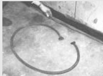
he simply slips the air-filled tubes in under the gap between the door and the floor. You could also fasten the tubes to the bottom of the door.
